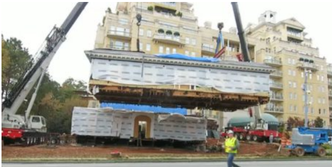
Workers prepare the two sections of the Randolph-Lucas House for relocation. Credit: Buckhead Heritage Society/Terry Kearns
